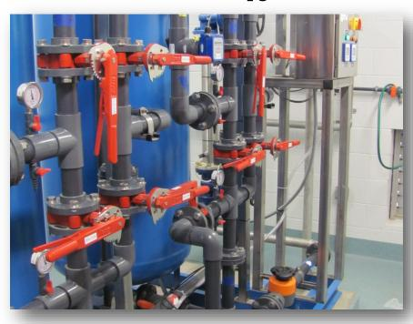
In 2016, HTWSA completed an upgrade to the Well No. 5 facility on Route 152. The Well had been out of service since the detection of arsenic in 2010. An arsenic removal system has been installed which is capable of reducing the arsenic levels in the treated water below the detectable limit. This system is similar to those already in service at the Well 1 and Well 2 Treatment Facilities.
